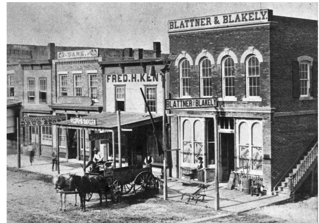
Figure 2.5 Images of the Town Top-Street scene in Junction City, Kansas. 1874. (Street scene in Junction City, Kansas) Bottom-Left-Junction City Courthouse. Built 1899. (Junction City Courthouse) Bottom-Right- Junction City Opera House. Built 1882. (Junction City Opera House)
