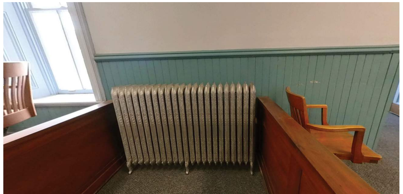
Existing radiator and beadboard wainscoting in the 2nd floor courtroom.
