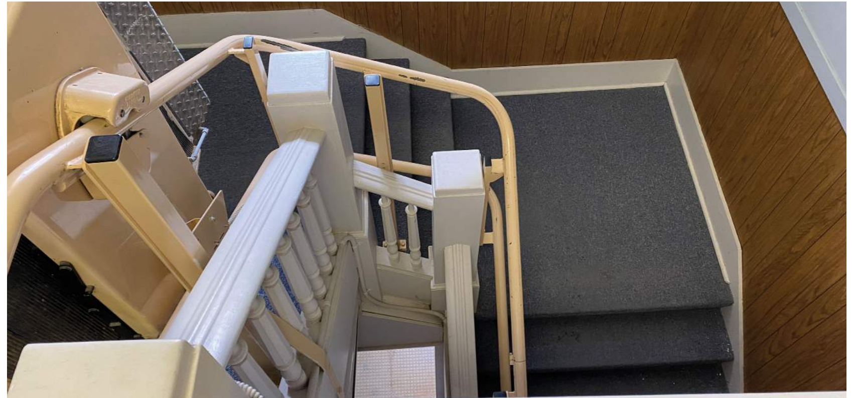
A chair lift was previously installed at the single open stair that connects the first and second floor.
