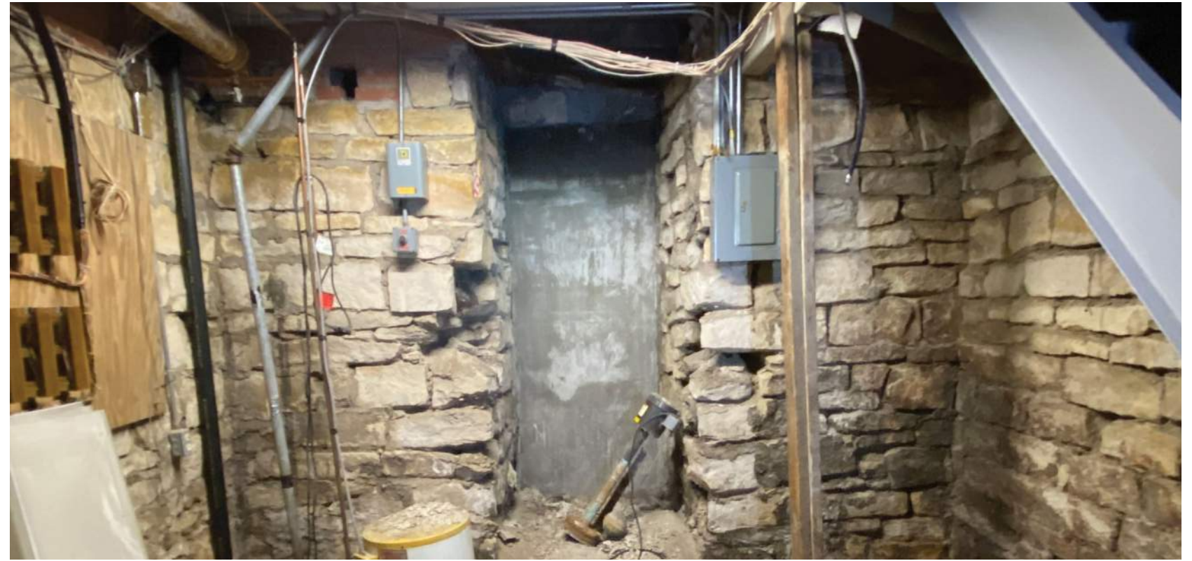
View of stone foundation walls in the excavated basement
