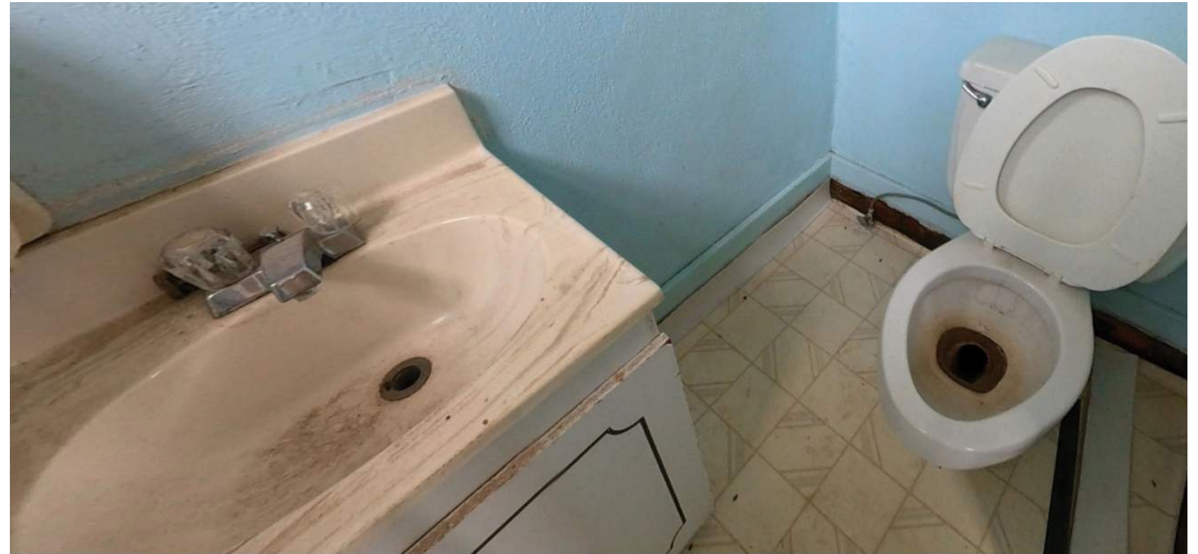
View of an inaccessible toilet room on the 2nd floor.
