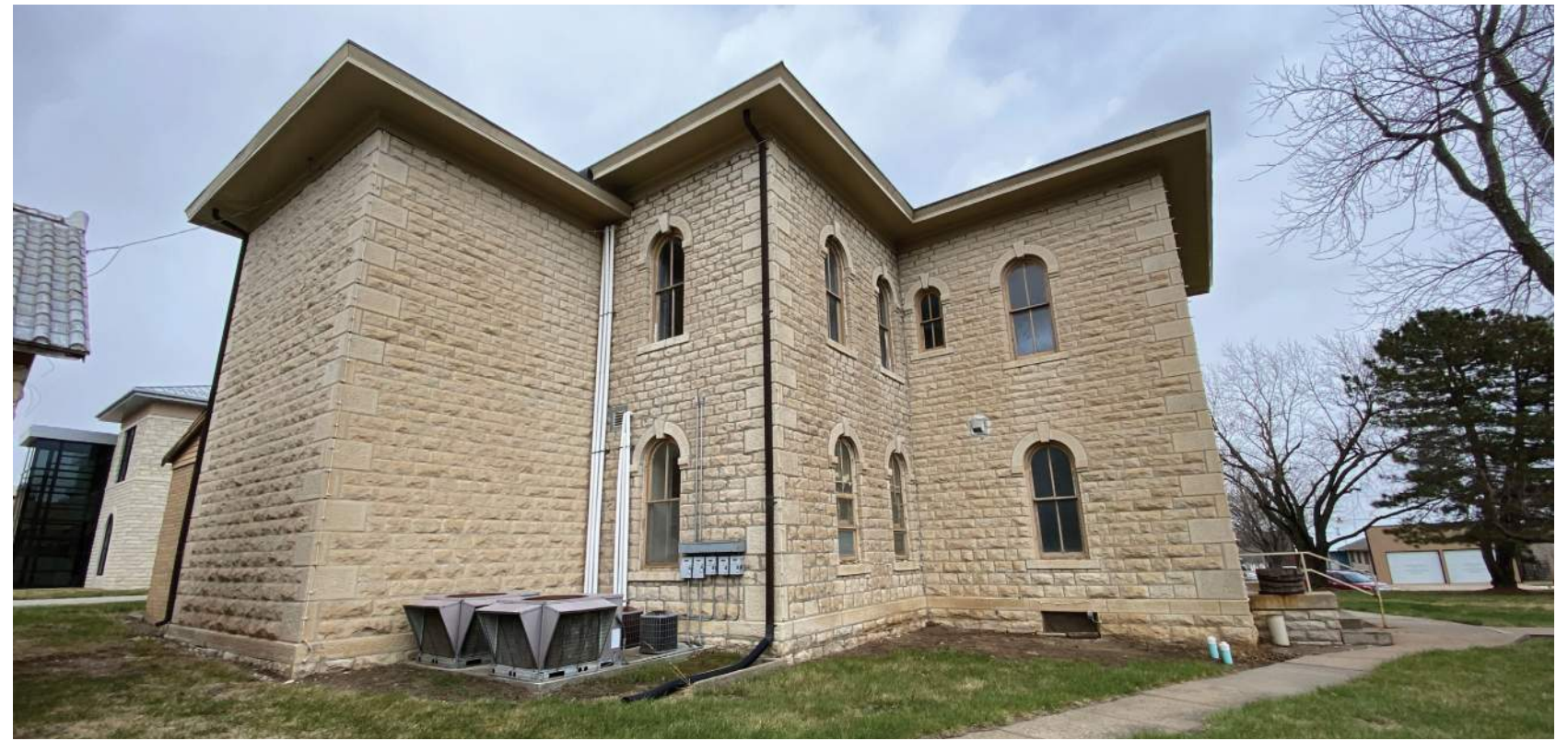
Previously installed mechanical and electrical systems are now outdated.
