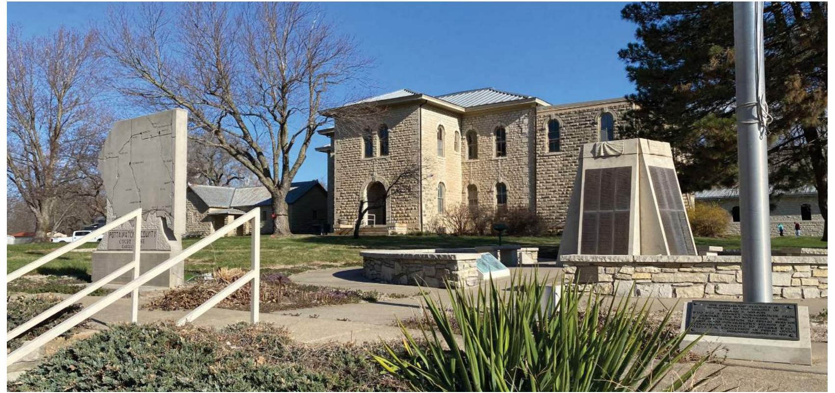
View of war memorial, flagpole, and stone monument at the corner of Main and N 2nd Street.
