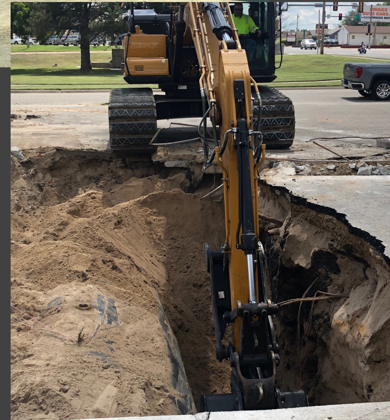
Underground Storage Tank Removal In Junction City
